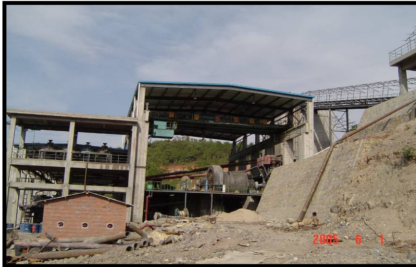
No.4 mill plant - 2,000 tpd
