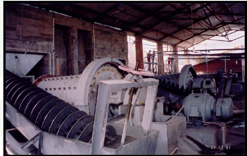
No.2 mill plant - 500 tpd
