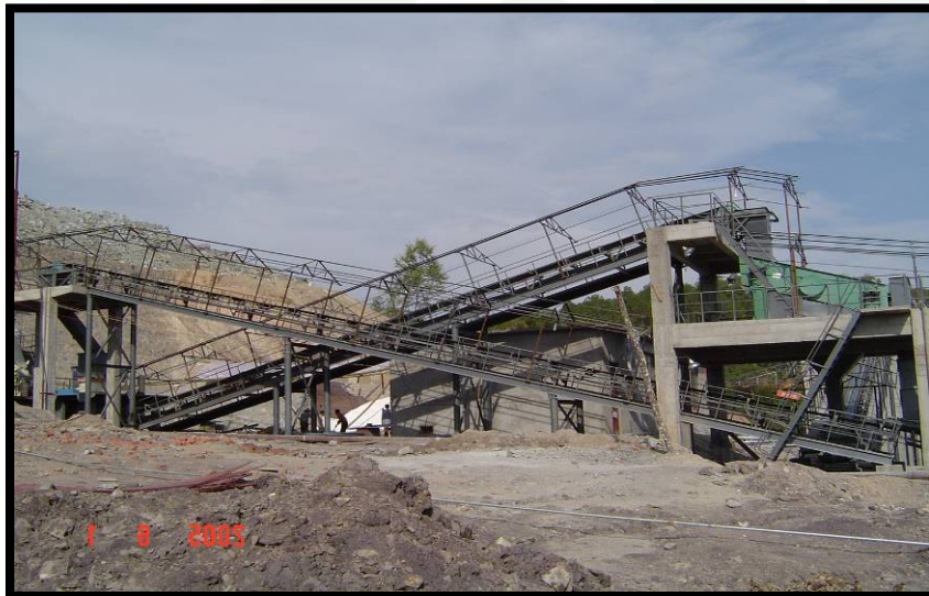
No.4 mill plant - 2,000 tpd
